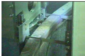
first cut on core shroud
