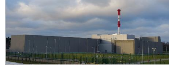
Low and Intermediate Waste Disposal (B25) – construction procurement
