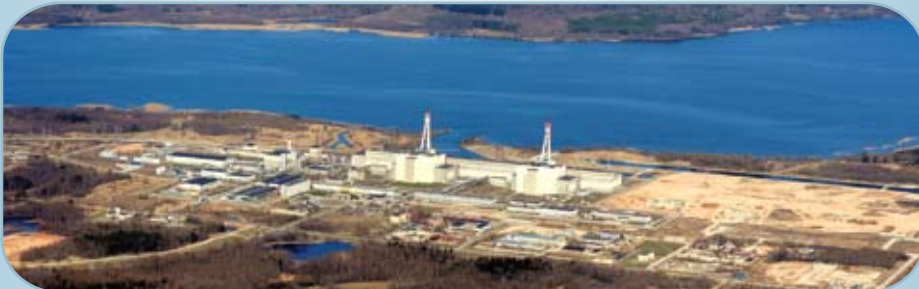
Do you know that on the INPP site there are about 150 buildings.
