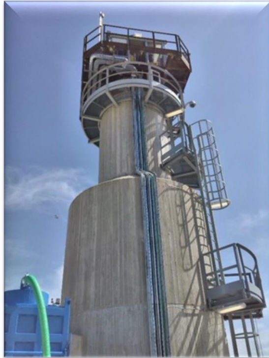
Mock-up of 12 metres high
