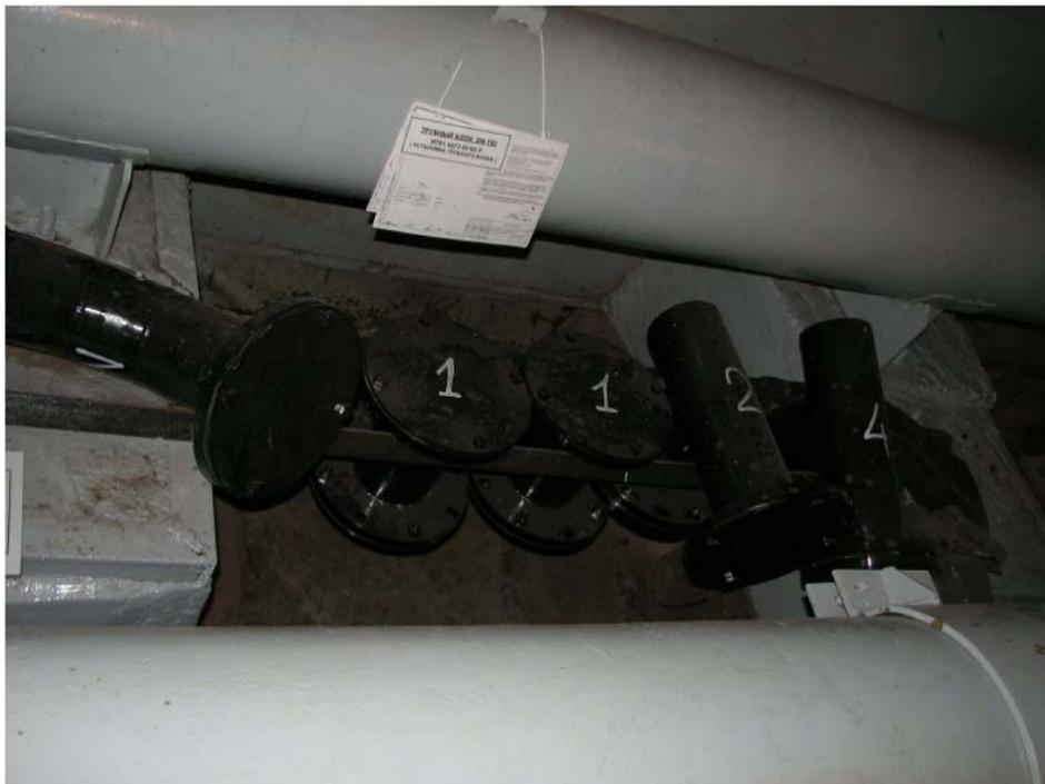
**Figure 8.4-3.** Pipe units DN 200 for modification МОД-05-02-716
