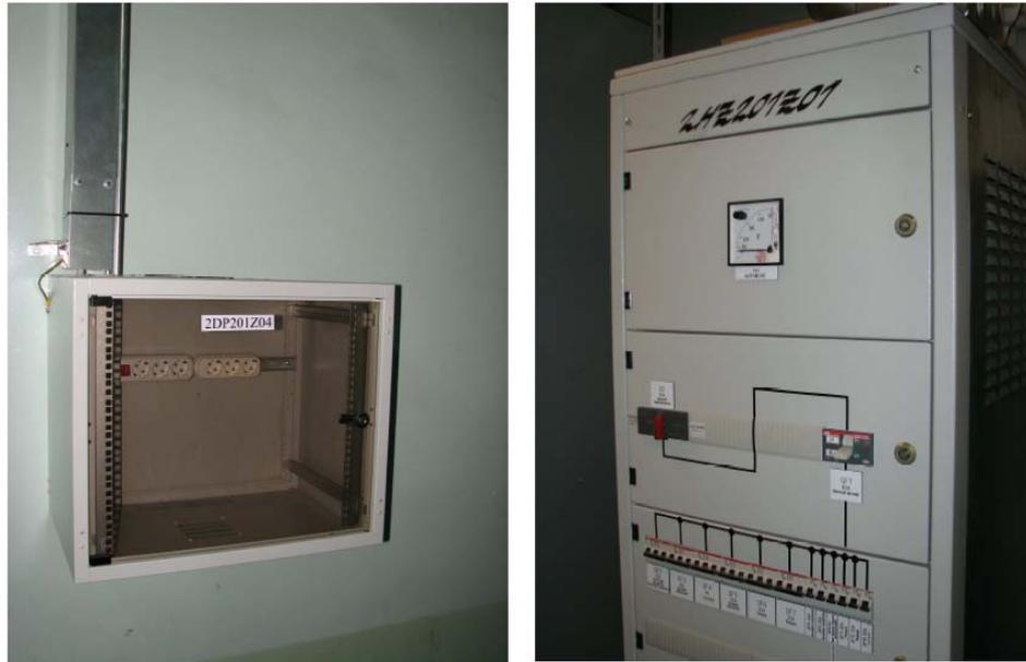
Figure 8.4-6. Portable accumulators charging board 2DP201Z04 and emergency switch cabinet 2HZ201Z01 in Room 2UPS-1
