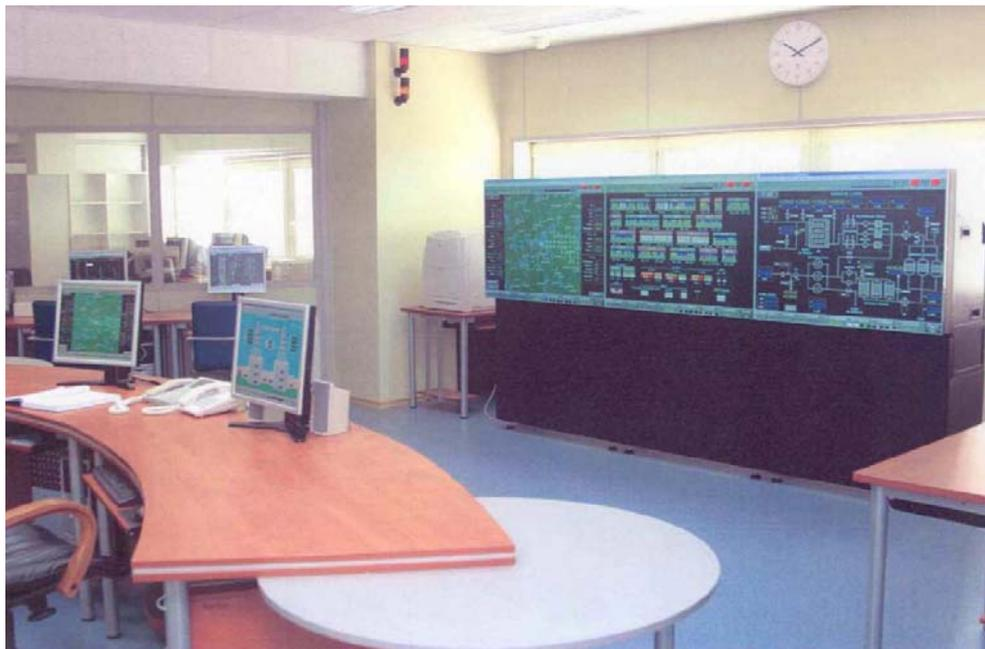
**Figure 8.4-15.** Radiation safety monitoring room with the automated radiation monitoring system means
