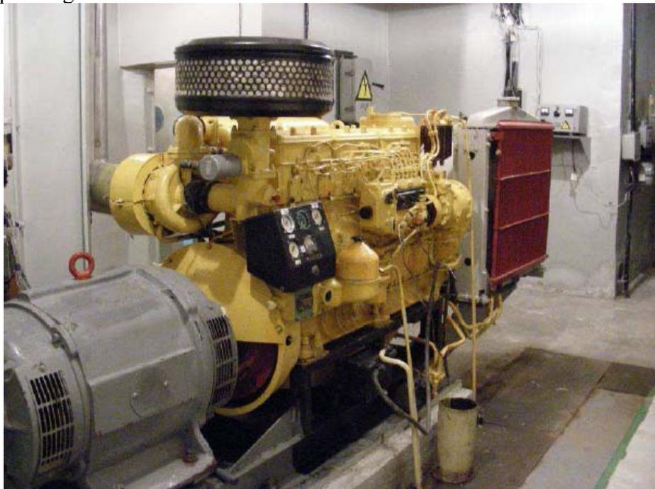
**Figure 8.4-14.** A stationary emergency diesel generator providing the OEP Accidents Management Centre in Bld. 185 functioning during the auxiliaries' blackout
