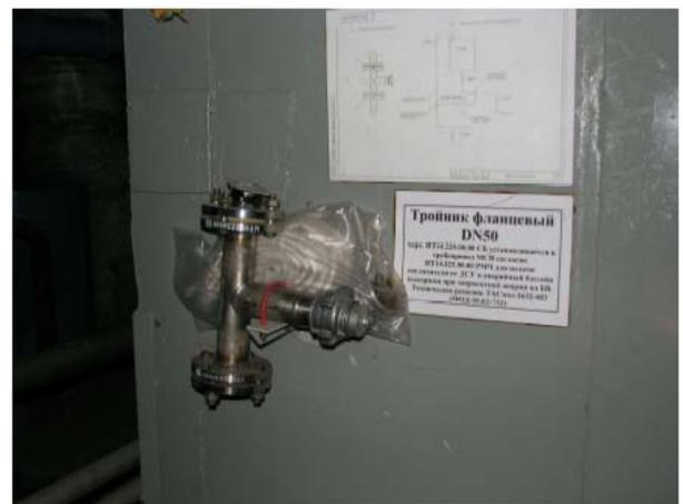
**Figure 8.4-10.** Pipe units DN 50 for modification МОД-05-02-732
