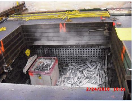
Good use of fixative application for dust and contamination control
