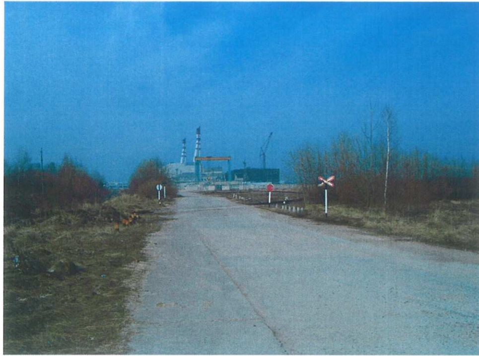
Figure 1. View from the east, on INPP Units 1 & 2, and partly built (abandoned) Unit 3.
