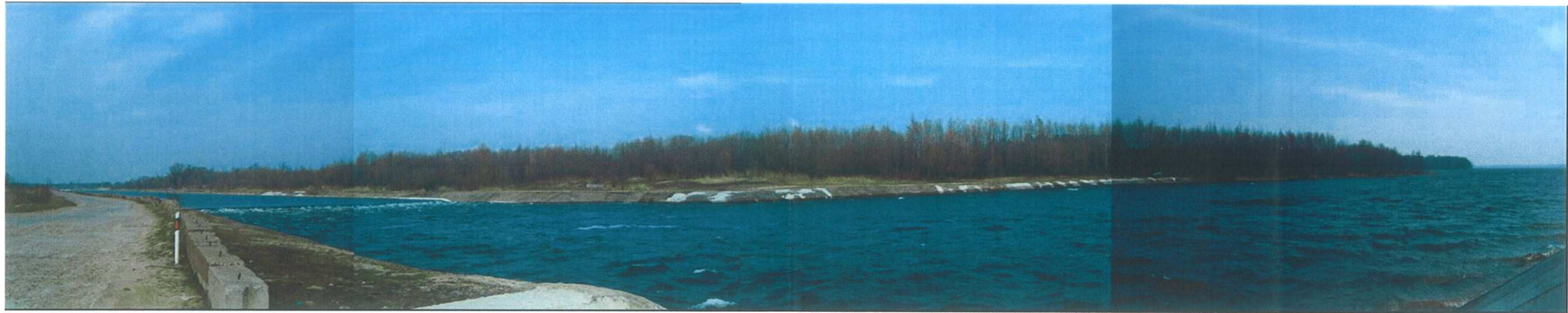
Figure 3. View on the warmed cooling water release and outtake channel
