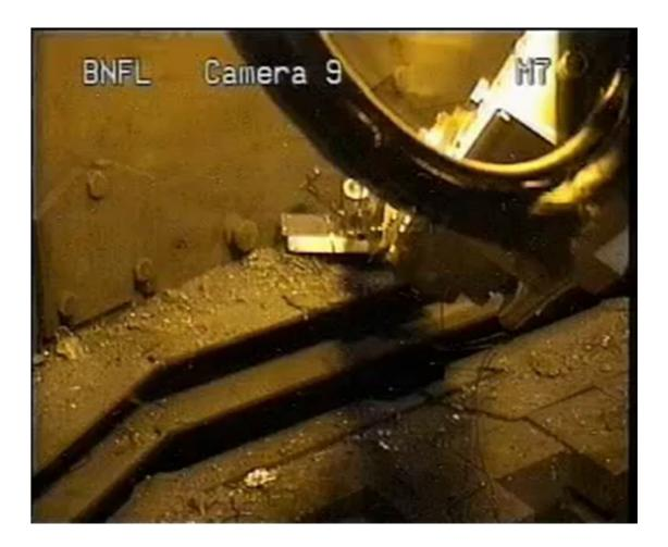
Layer 1 Gas seal debris – needed to be cleared prior to deploying a plasma cutting head to section
