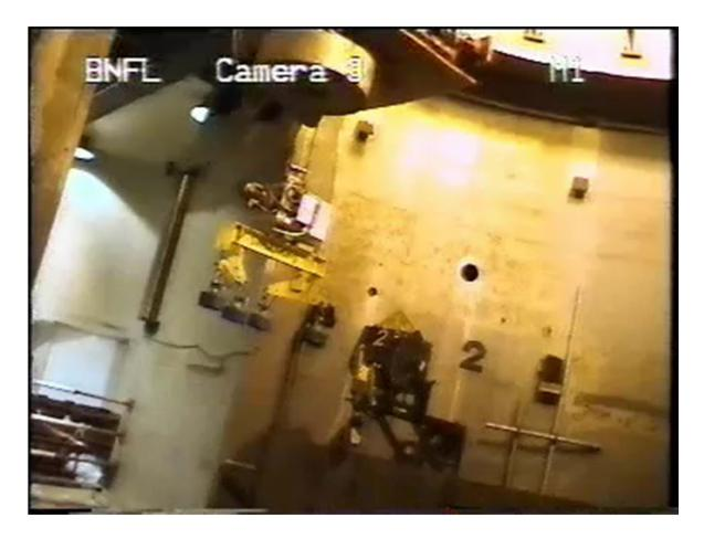
Steel core support plates – highly activated. Removed after all bearings, arrestor mechanisms and residual op waste in the housings dealt with
