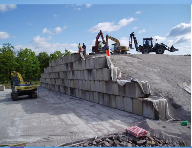
Installation of the temporary protective wall
