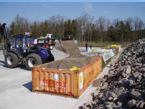
The container is filled with sand. Sand is levelled and compacted
