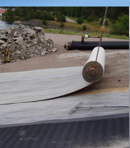
The levelling layer is covered with insulation layers — bentonite carpet and HDPE geomembrane
