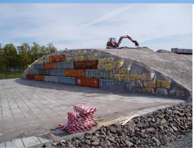
After the forming of the stack, a levelling layer is formed which is the basis for the insulating layers
