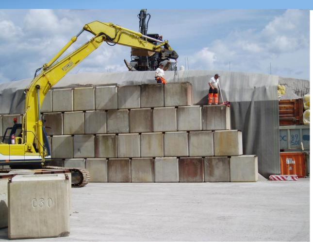
Installation of the protective wall from concrete blocks
