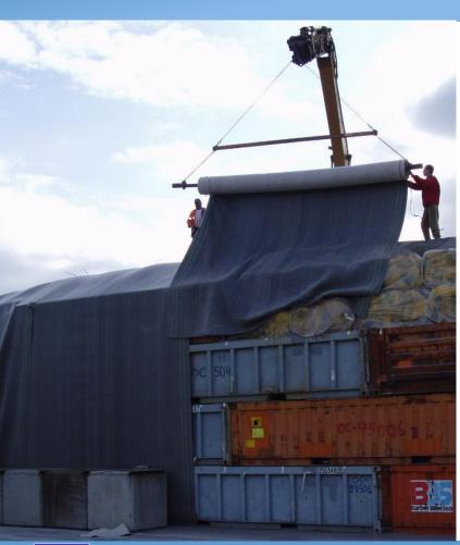
Installation of vertical insulation - bentonite clay carpet
