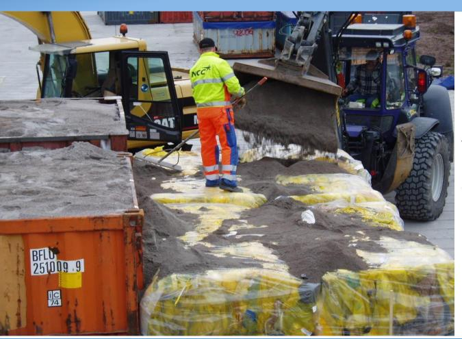
The spaces between the "small" packages are also filled with sand
