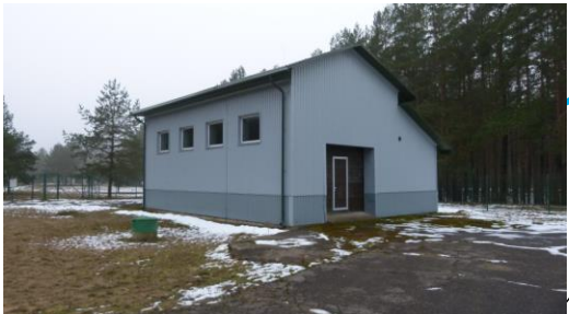
The former decontamination building
